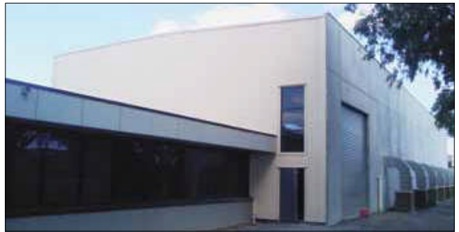
Outside completed additional plant
