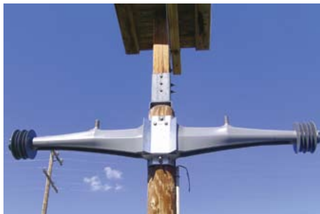
Integrated cross arm insulator and universal mounting with North American Raptor nest above.
